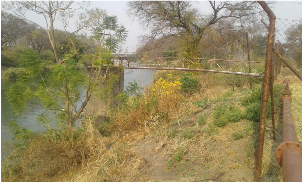
Picture 10: Mupfure Raw Water Abstraction Plant
