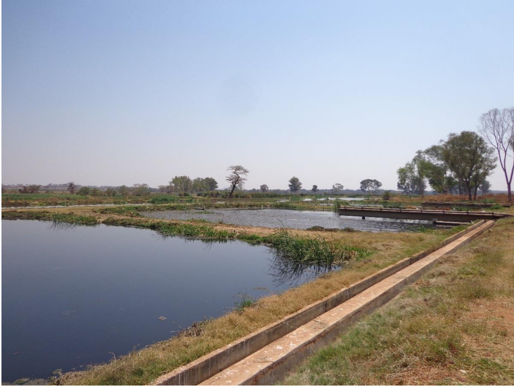
Picture 20: ZMDC sewage ponds
