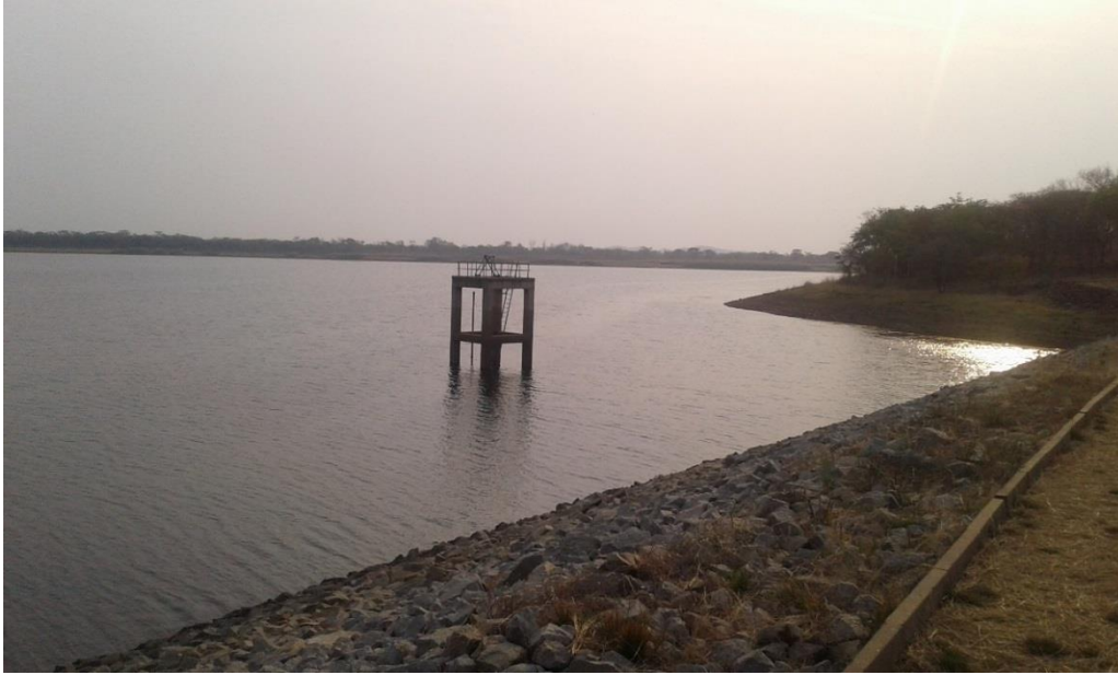
Picture 11: Clifton Dam
